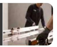
A cutting guide fitted with a diamond tip tool is recommended.
