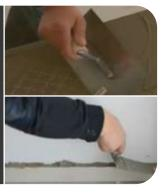
Wipe the grout lines in a circular motion with a sponge and water to set the grout just below the tile surface. Follow up with a grout haze remover to clean the tile.
