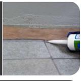
Wait approximately three weeks for the grout to cure completely before sealing the grout.
