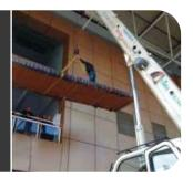
Where possible, mechanical lifting systems should be used for delivering slabs above the ground floor.
